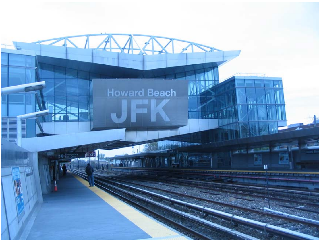
Howard Beach station – subway platforms and Airtrain connector bridge
