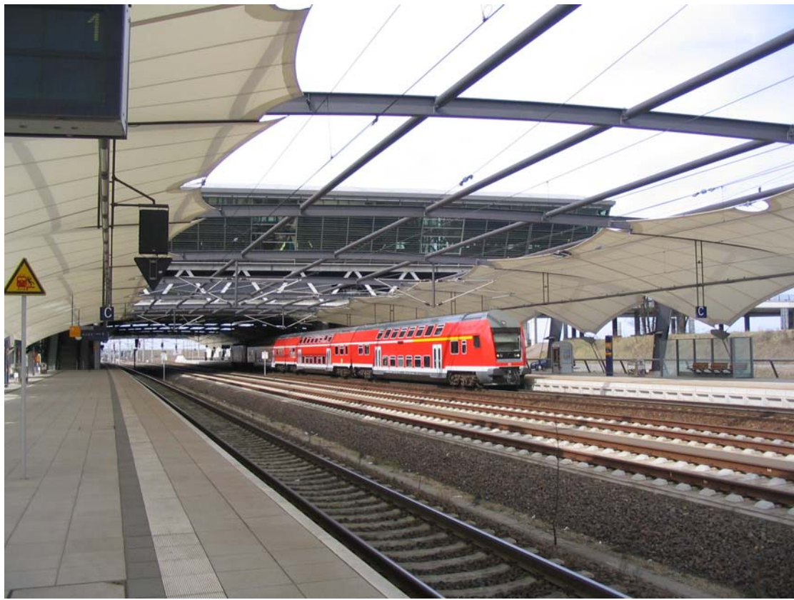
Leipzig-Halle airport station, showing check-in area above the platforms.
