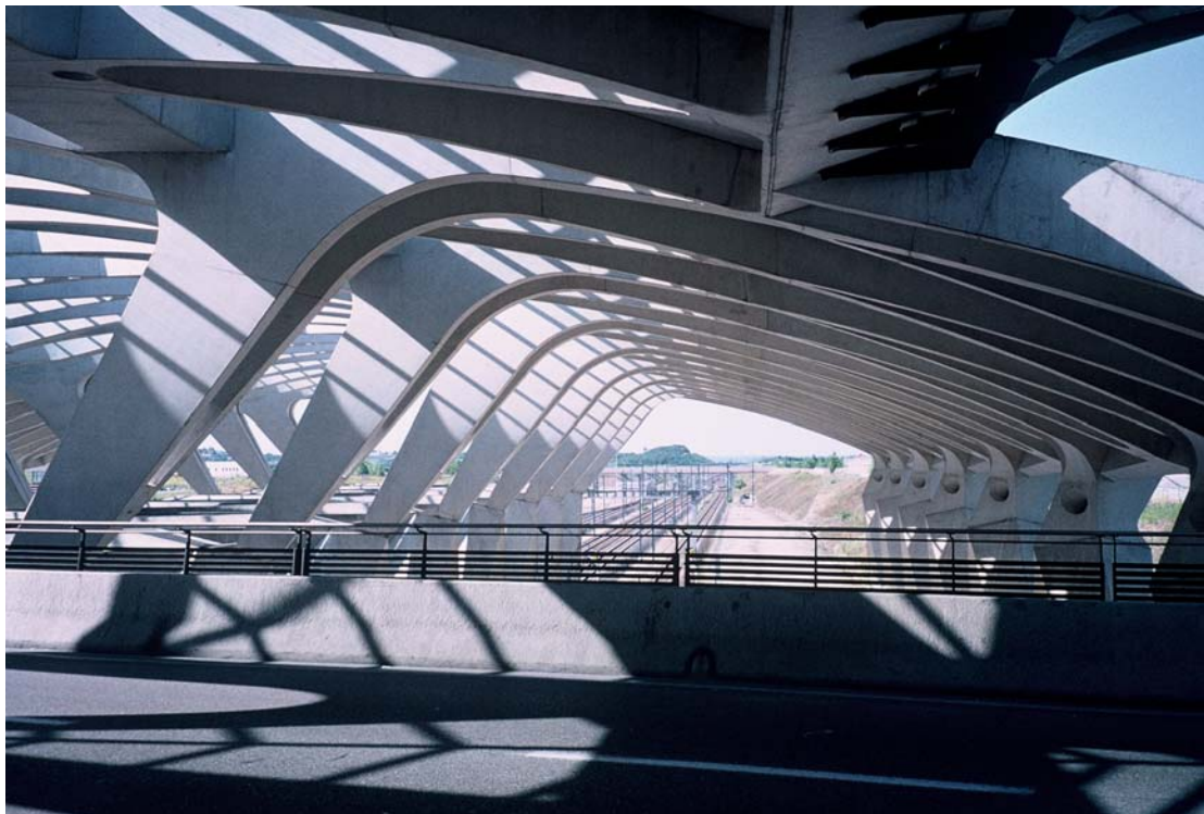
Lyon St-Exupéry station
