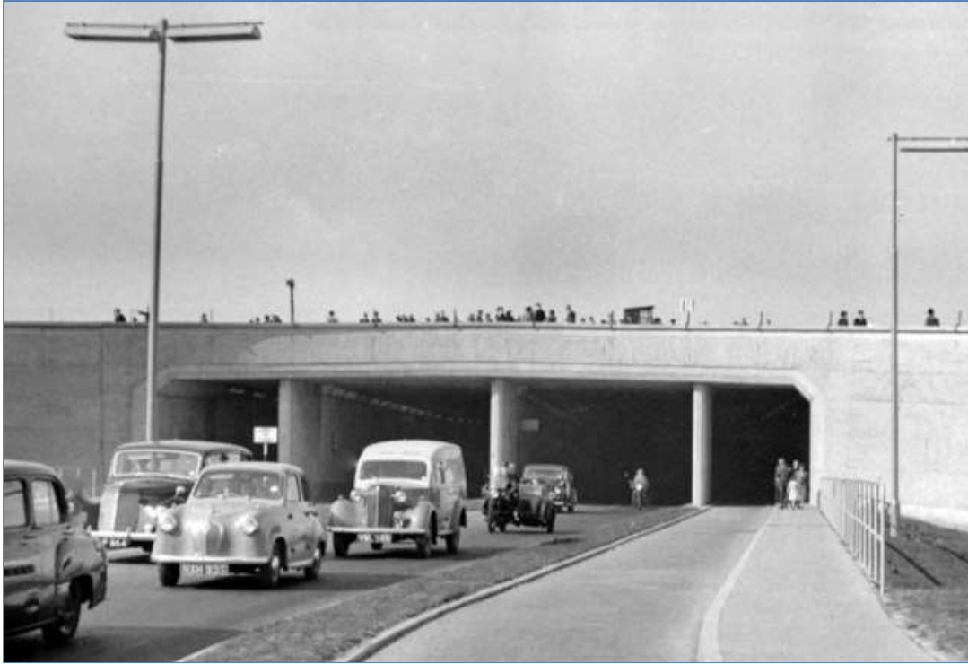
Figure 2: London Airport road tunnel 13
