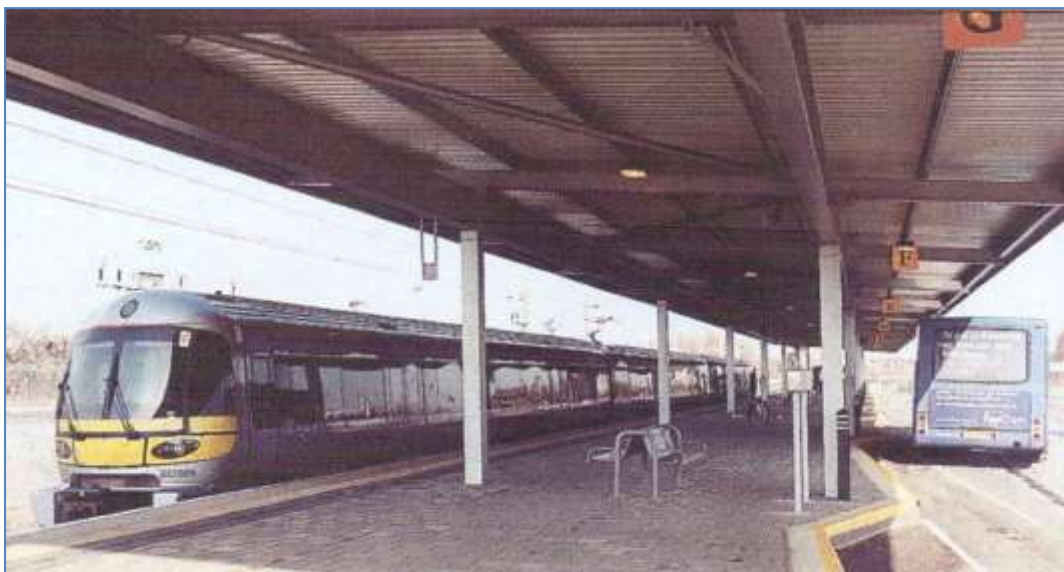
Figure 10: Fast Train temporary station
